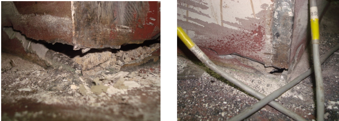
Figure 9: Fracture of West Column (North West Corner) at 2.7% Drift
